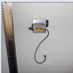
Converter/Battery Charger
