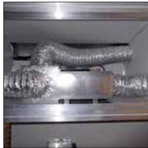
34,000 BTU Furnace w/ Thermostat
